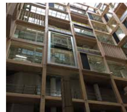
ANCHORAGE PLACE ATRIUM
